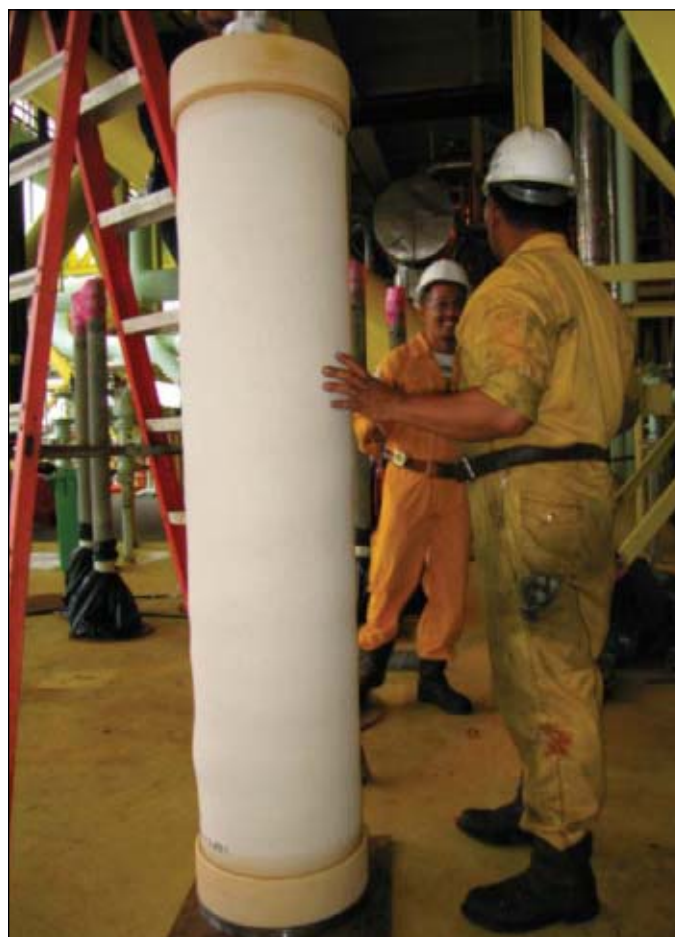
This photo shows one of the 16-in. membrane elements before being installed in its individual enclosure (Fig. 7).
