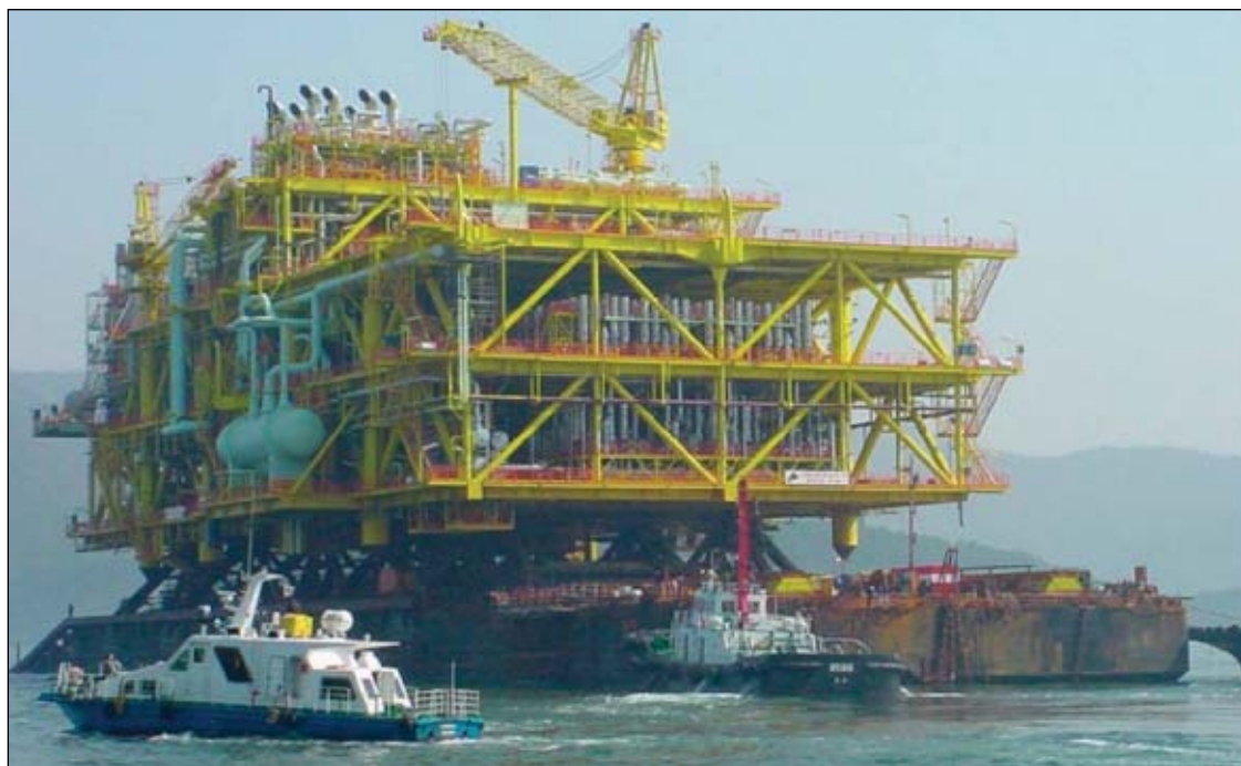
The Cakerawala production platform is moved into position in the Gulf of Thailand (Fig. 1).
