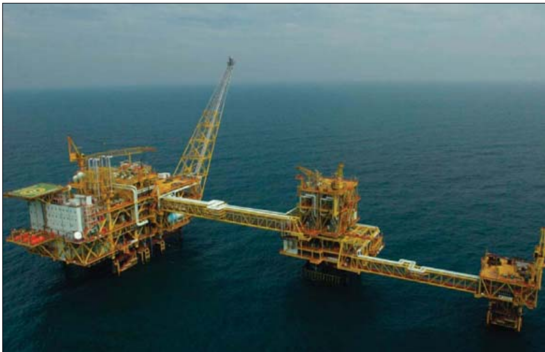
The Cakerwala production facility can produce 425 MMscfd of sales gas with a final CO 2 specification of 15% (Fig. 2).
